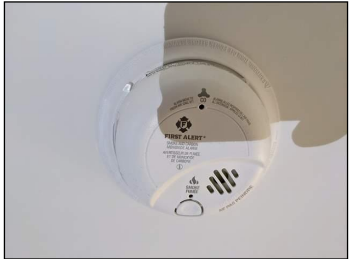
106. Combination smoke/CO alarm(s) noted
