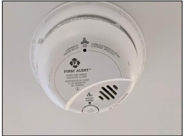
104. Combination smoke/CO alarm(s) noted
