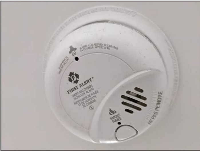
103. Combination smoke/CO alarm(s) noted
