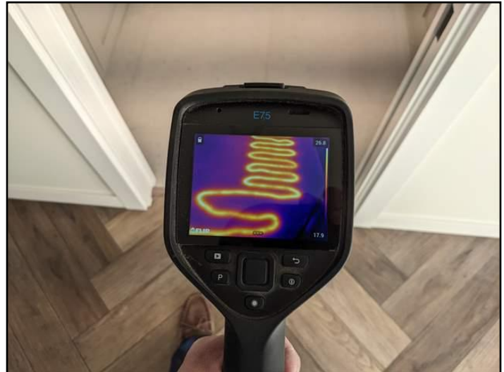
127. Electric radiant heat
