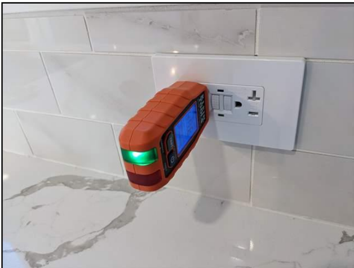
91. GFCI - bathroom and exterior
