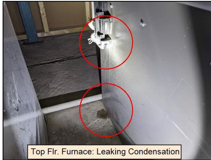
145. Condensate leak
