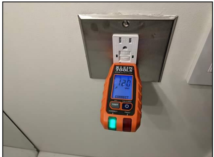
90. GFCI - bathroom and exterior
