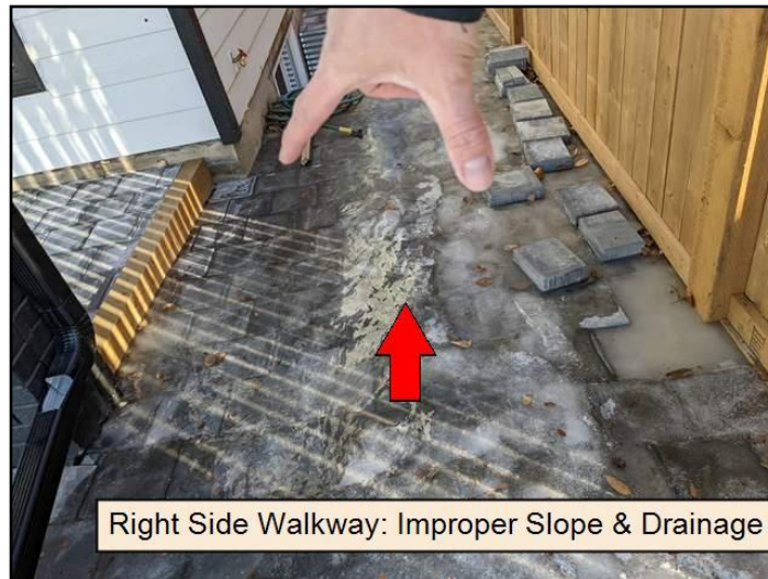
3. Improper slope or drainage
