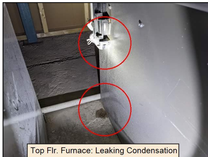
6. Condensate leak
