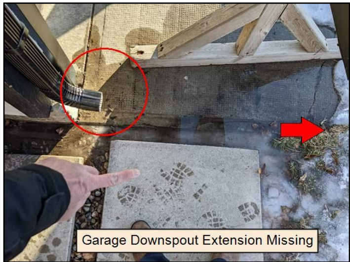
74. Discharge too close to building
