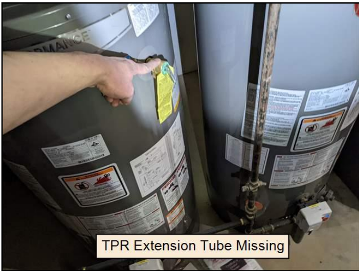
163. Discharge tube missing
