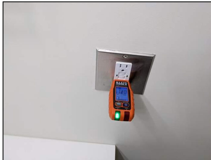
93. GFCI - bathroom and exterior
