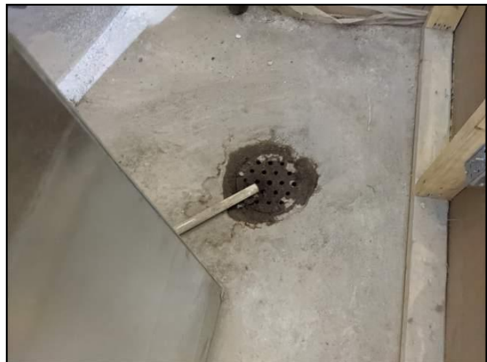
159. Near heating system
