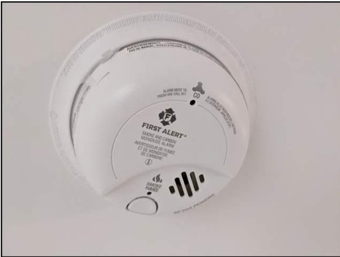
105. Combination smoke/CO alarm(s) noted
