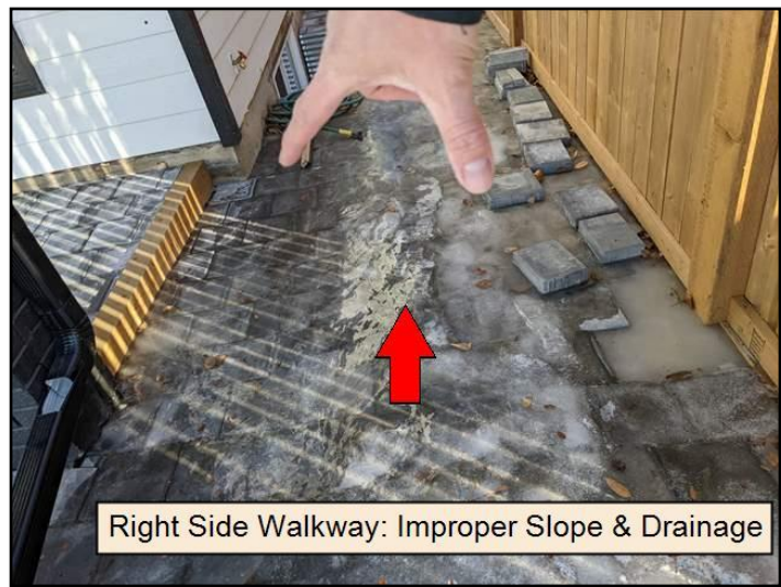
76. Improper slope or drainage
