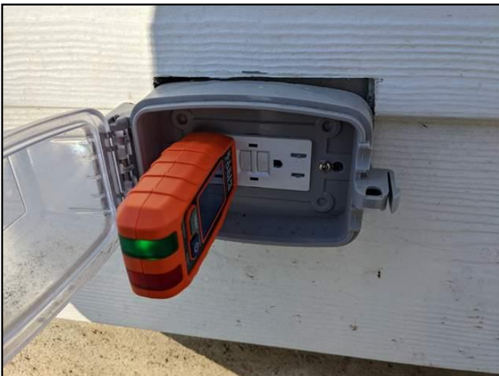
89. GFCI - bathroom and exterior
