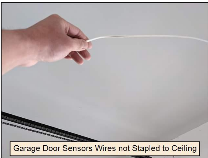
Garage Door Sensors Wires not Stapled to Ceiling
