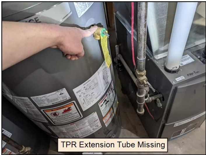
164. Discharge tube missing
