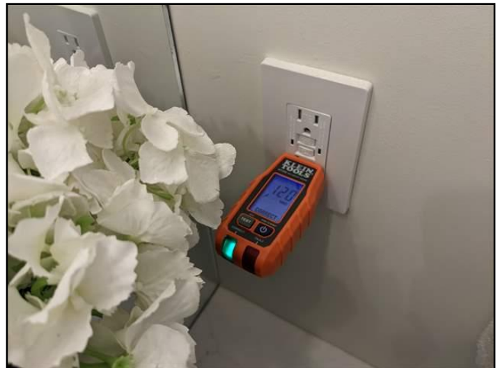
92. GFCI - bathroom and exterior
