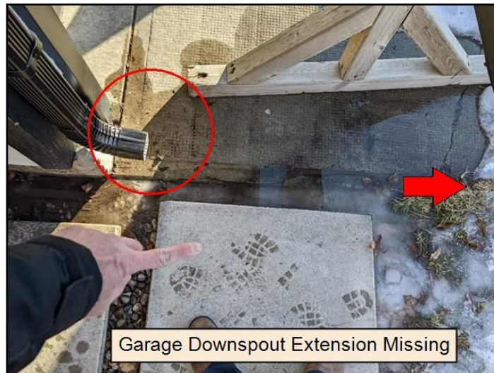
1. Discharge too close to building
